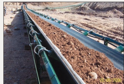
Complete Canning Field Conveyor Bays (900mm belt - steel safety handles - in 2.6m long bays).
