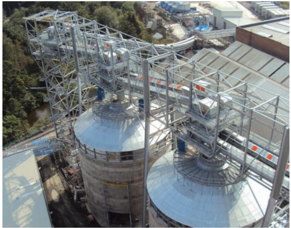
undersize chutes of the disc screens (by others) before elevating via heavy duty lattice gantries to a height of approximately 30 metres, before discharging at the top of transfer tower A.
